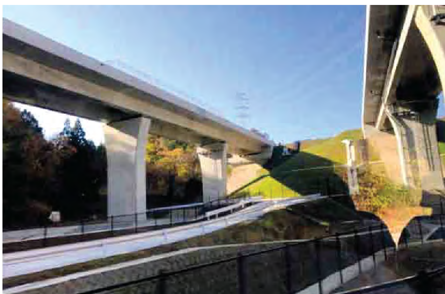
Figure A 2: Shin-Meishin Expressway
