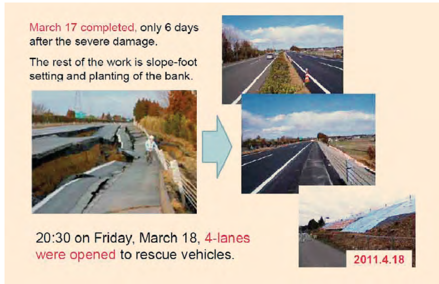
Figure 7.18: Recovery example – Naka repair
