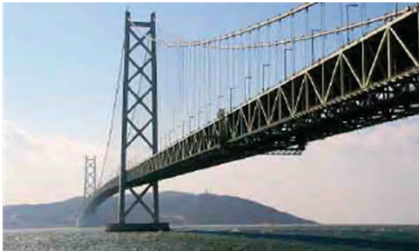
Figure A 4: Akashi Kaikyō Bridge
