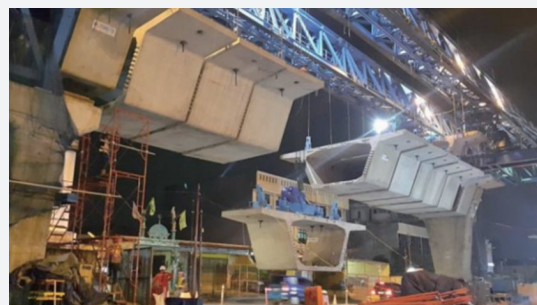
Figure 8: Segmental box girder of Pettarani elevated toll road
