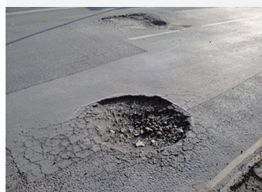
Figure 2: Pothole
