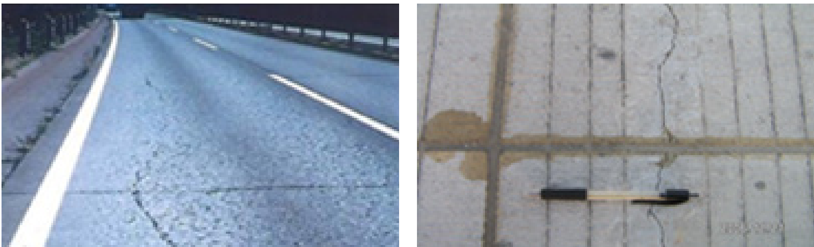
Longitudinal cracking Transverse cracking
