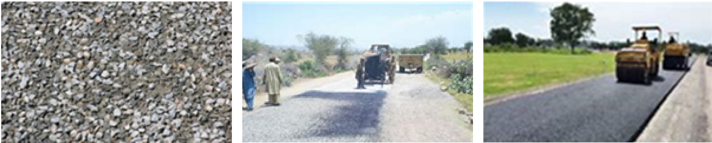
Examples of double bituminous surfacing treatments (not including sprayed/chip seals)
