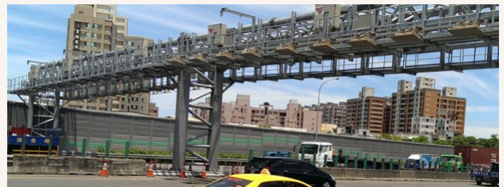
Electronic Toll Collection System on Taiwan’s National Highway
