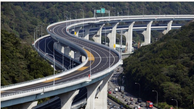
National Freeway No. 1 Widening Project— Wugu to Yangmei Section
