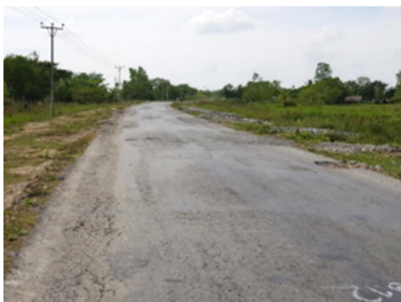
Figure 6: Site before trial
