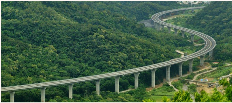
Elevated Highway in Anshuo to Caopu Section of the South Link of Taiwan Provincial Highway No. 9
