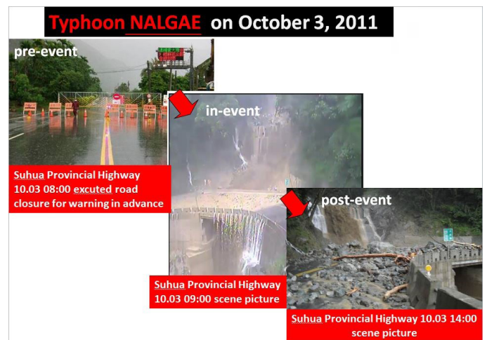
Figure 7: Images of hazards after road closure induced by heavy rainfall
