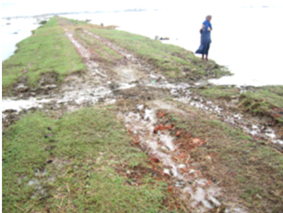
Figure 2: Normal condition of a rural road
