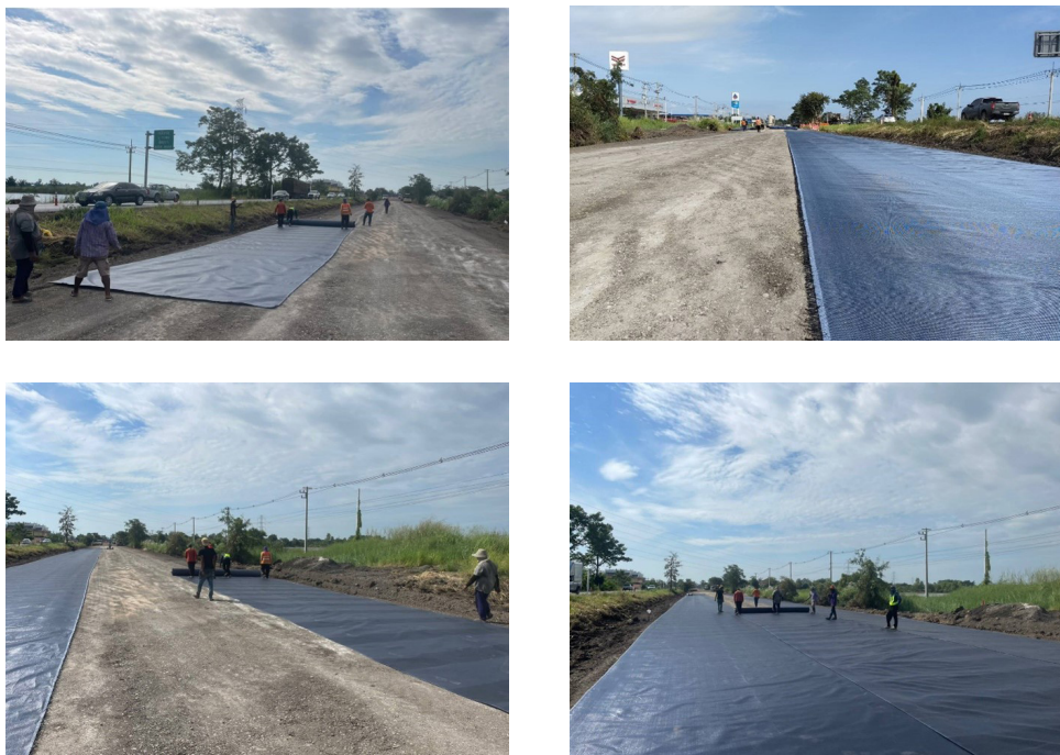
Figure 5: Installation of woven geotextile TenCate Mirafi® H2Rx
