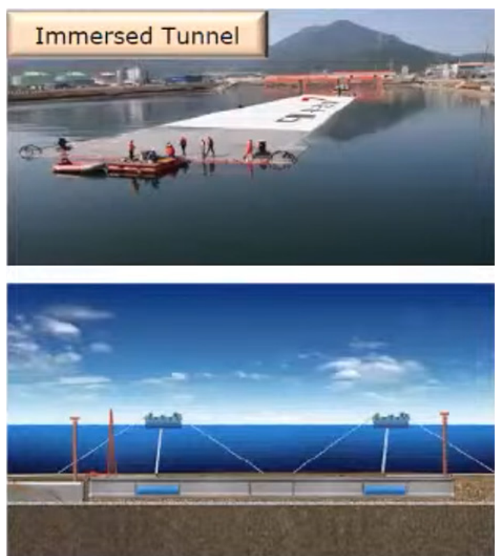
Figure 1 Immersed Tunnel Construction
