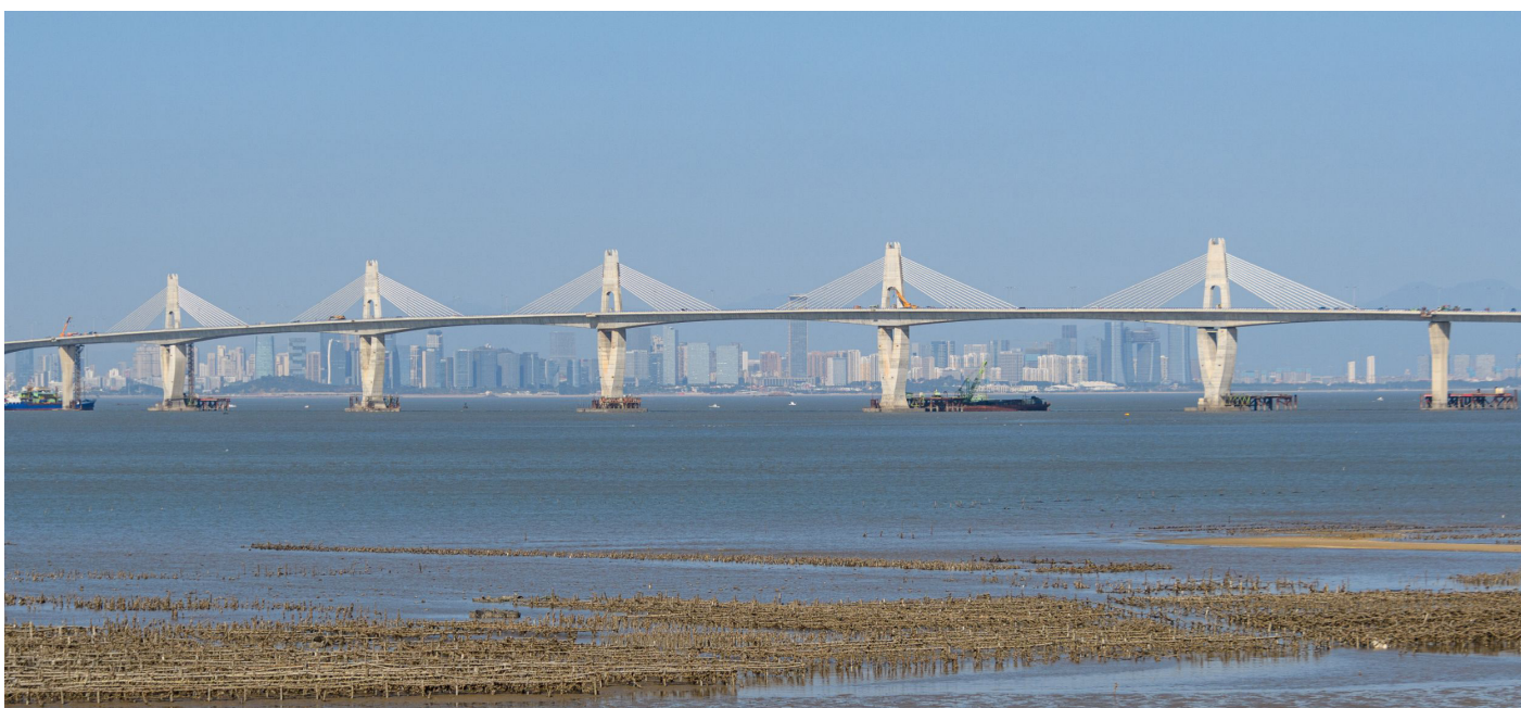
Figure 14: Joining of the Kinmen Bridge 2022.07.22
