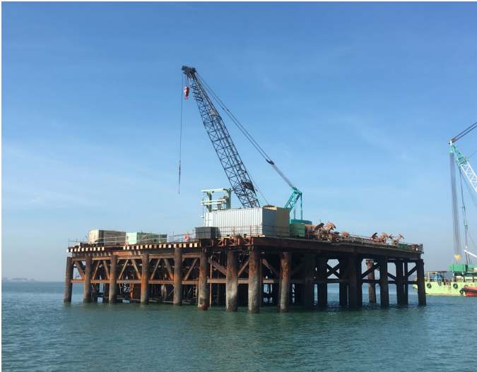
Figure 4: CASE 1 Build the Construction Platform with the Jacket Steel Pipe
