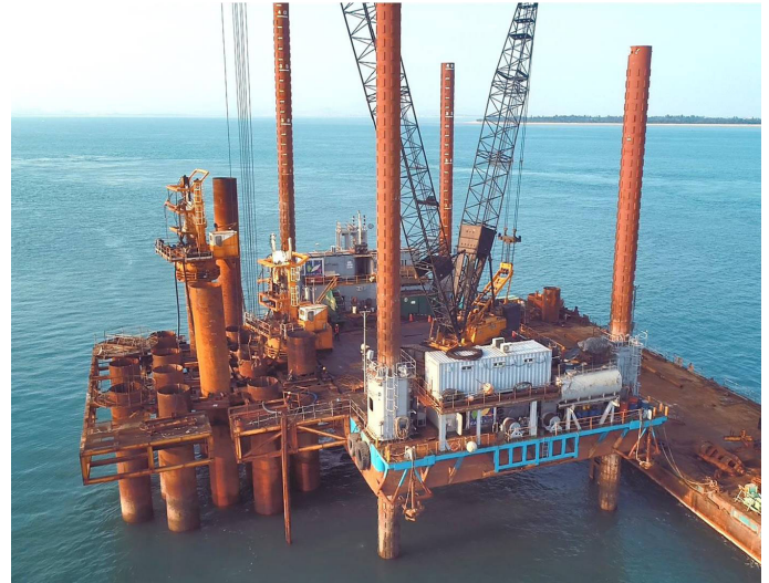
Figure 5: CASE 2 Use Jack-up Platform Ships as Gantry
