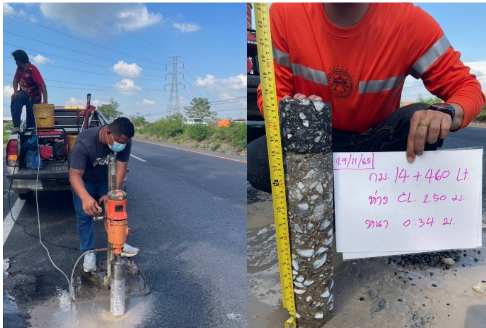
Figure 7: Extraction of 100 mm diameter core
