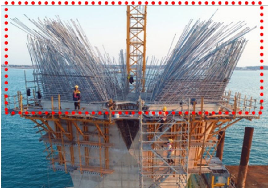
Figure 12: The main reinforcement has a large amount of connections with various rotation angles
