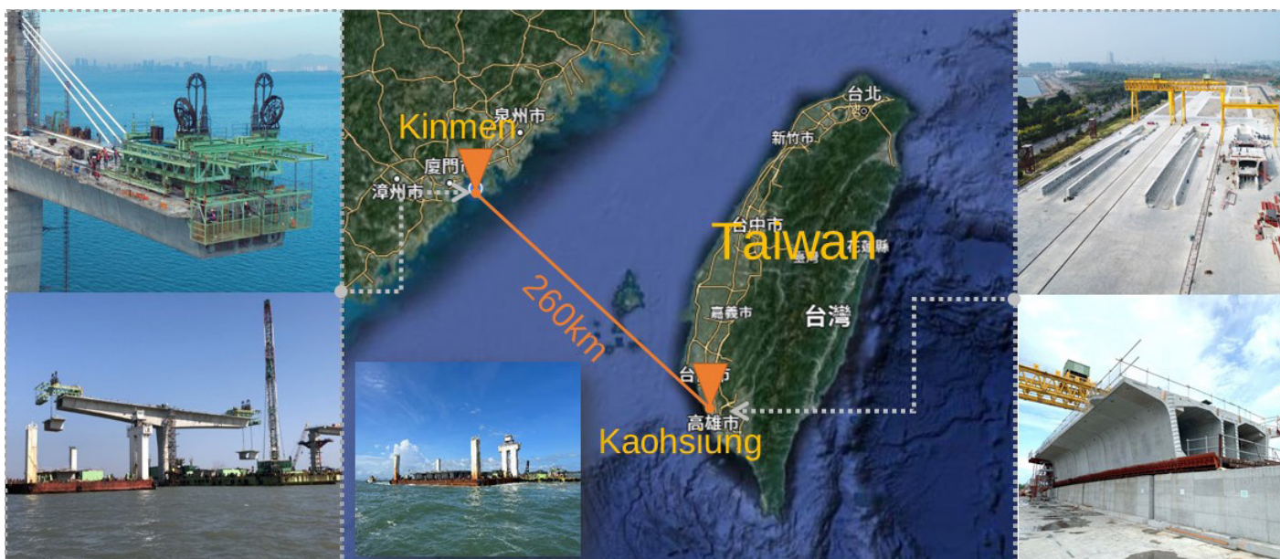
Figure 13: Production, Transportation and Hoisting of Segmental Precast Box Girder
