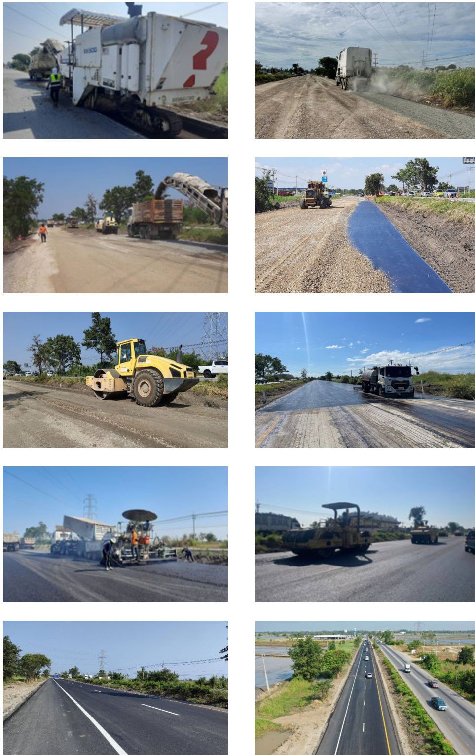
Figure 6: Construction process
