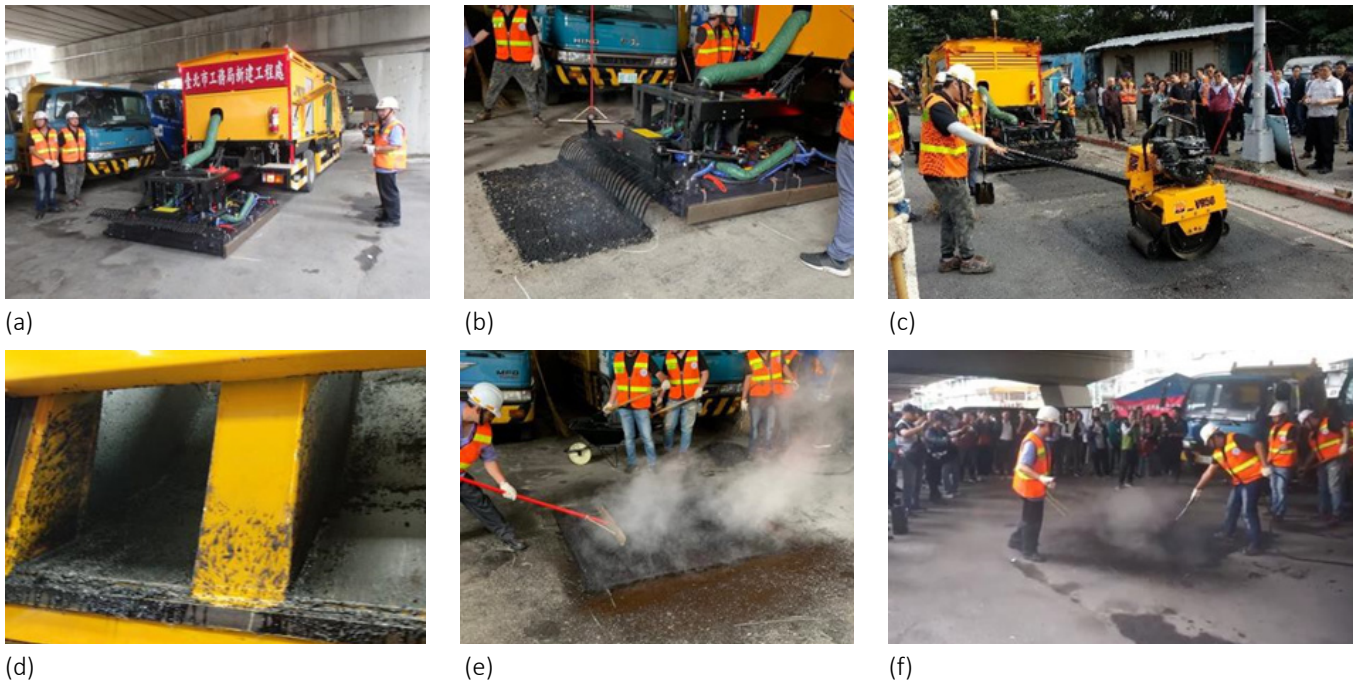
Figure 5: Hot-in-place recycling repair unit PM220 operation process
