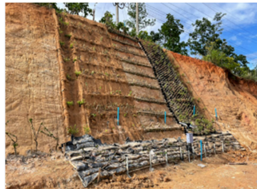
After construction 2022- July
