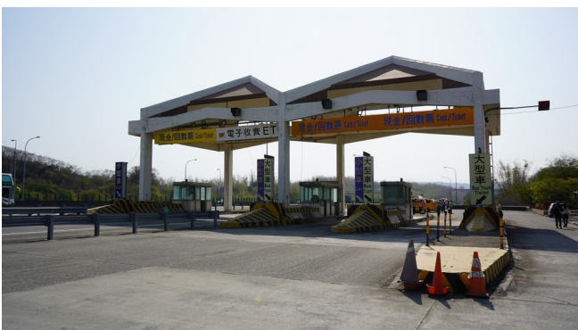
Manual Toll Booth has become a thing of the past
