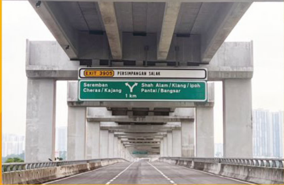
Elevated highway at SPE
