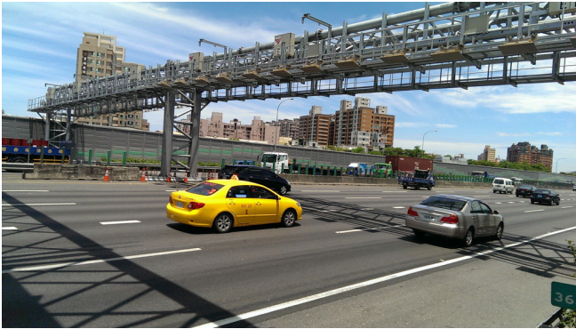
Taiwan MLFF Toll Gantry
