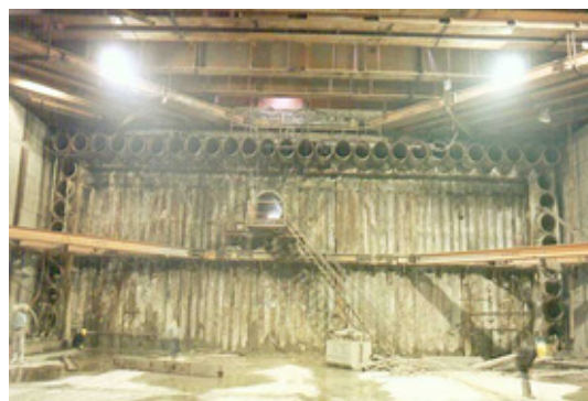
Underground tunnel size and pipe roof around the tunnel
