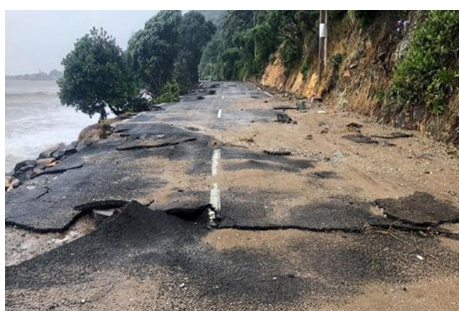
Figure 3: Disruption caused by storm surge to the SH network on the Coromandel Peninsula
