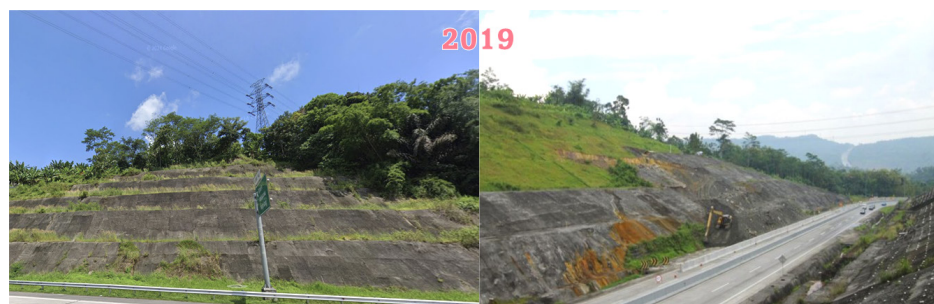
Figure 3: Slope remedial measures using shotcrete and bolt at Toll Road Semarang-Bawen: (left) successful work, (right) unsuccessful work
