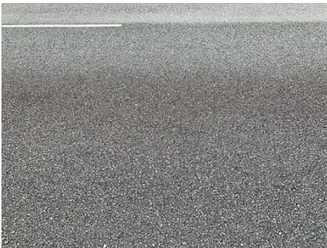
Figure 11: No visible defects on APFMA test section (March 2024)
