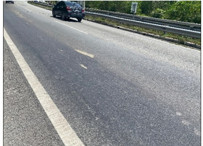
Figure 10: Block cracking in control mix (March 2024)
