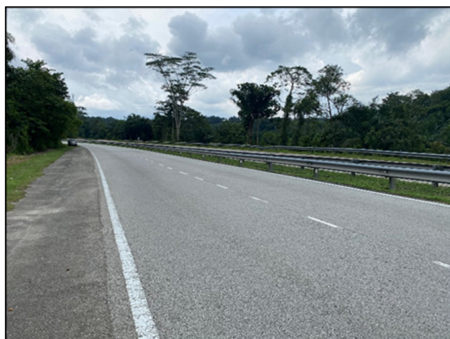
Figure 4: SFM after 6 years of service in Perak, Malaysia
