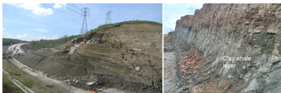
Figure 2: Slope failure at Toll Road Semarang-Bawen, Central Java, Indonesia
