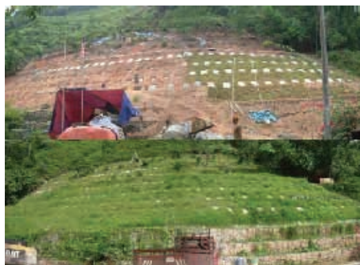
Figure 11.3: Use of plastic sheets to prevent slope erosion
