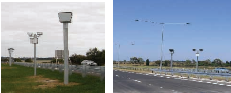
Figure 8.6: Point-to-point camera system on the Hume Highway
