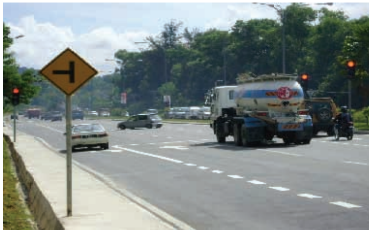
Figure 8.14: Typical example of U-Turn metering in Sabah
