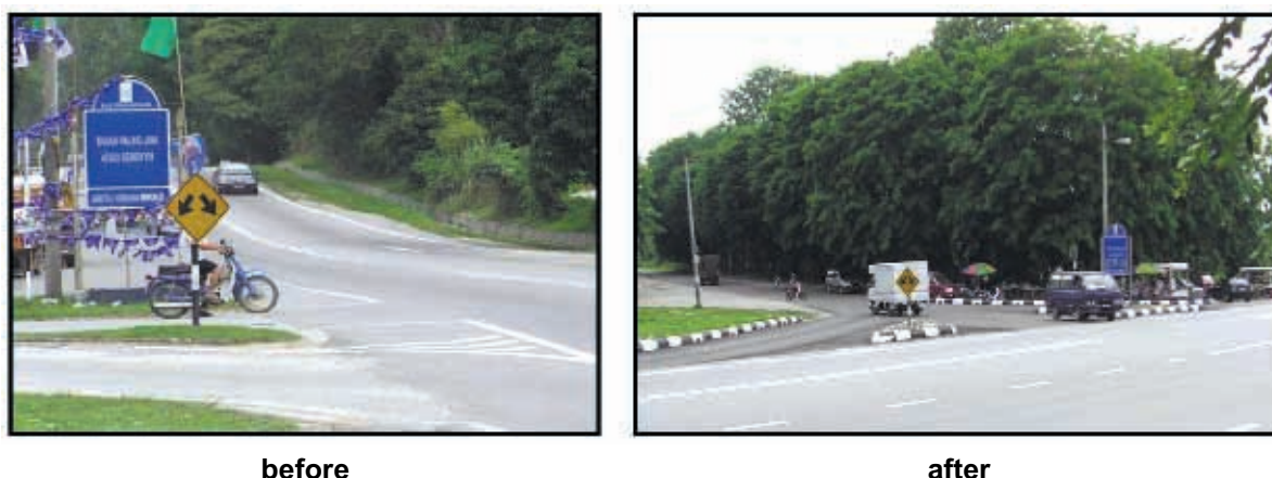
Figure 10.3: Example of improvement to a road junction
