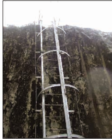
Figure 11.5: Typical cascade drain with hand railing
