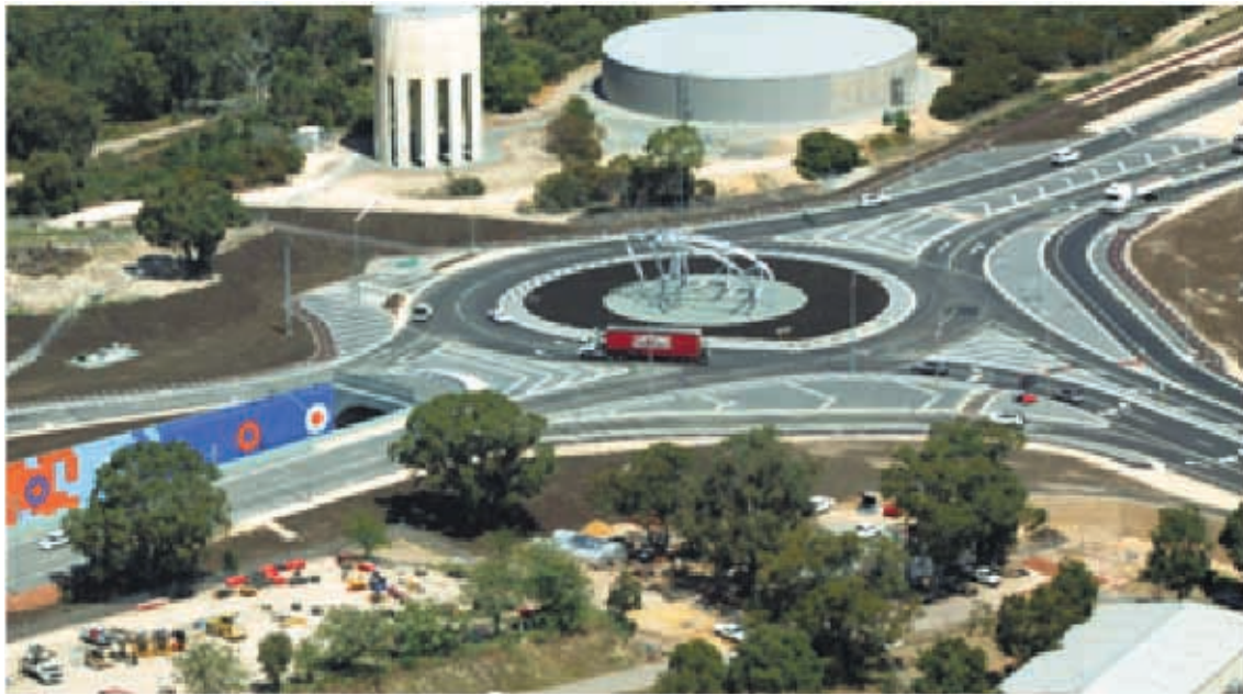
Figure 11.1: Mandjoodoorgap Drive–Mandurah Road intersection adjusted from traffic signals to a roundabout, which enabled signature public art to be installed
