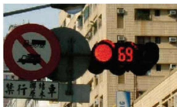
Figure 8.13: Built in count down monitor for red light (red figure)
