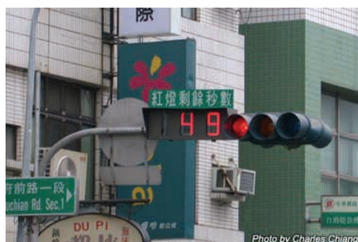
Figure 8.11: Plug in count-down monitor for red light (red number)
