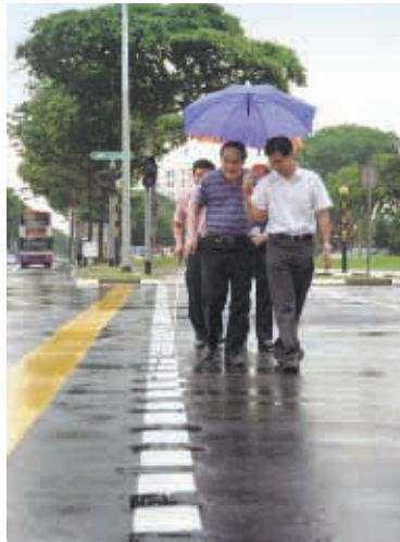
Figure 6.10: Crossings with dashed lines are safer for the visually-impaired
