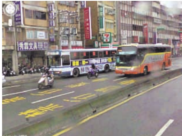
Figure 5.5: Roosevelt Road has no bus exclusive lanes and buses interfere with other vehicles
