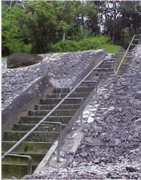
Figure 11.4: Typical vertical ladder on a rock slope
