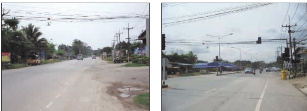
Figure 11.14: Road conditions on SR3348 before (left) and after (right) improvement
