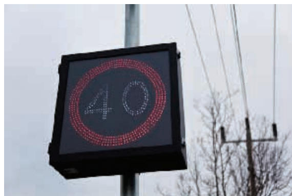
Figure 8.3: Electronic variable speed limit sign
