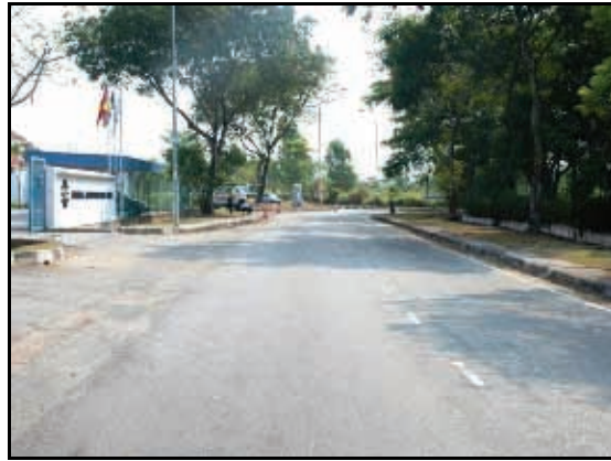
Figure 7.11: Absence of warning signs – view from Jalan Ijuk 26/5
