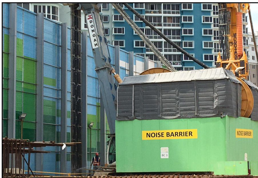
Localised noise encapsulation for heavy machinery
