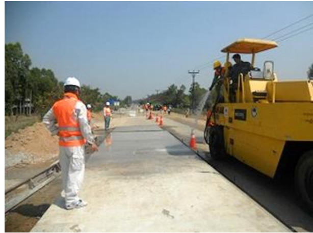
Figure 50: Secondary curing
