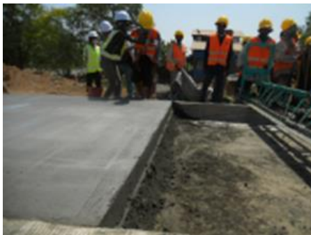
Figure 47: Construction joint
