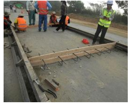
Figure 43: Fixing the dowel bars with forms
