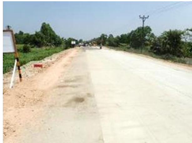
Figure 52: Pavement after the project
