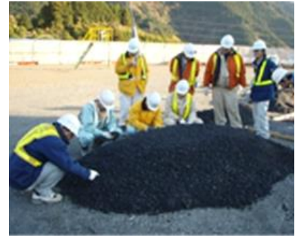
Figure 26: Trial mix at plant
