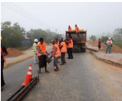
Figure 38: Setting of the forms
