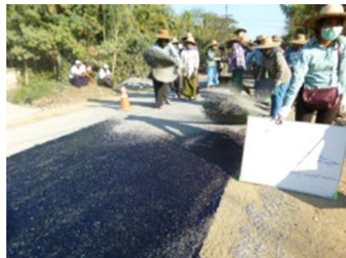
Figure 11: Spreading aggregates
