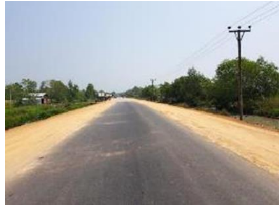
Figure 31: Site after trial
