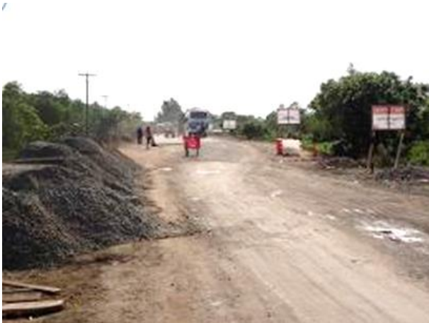
Figure 51: Pavement before the project
