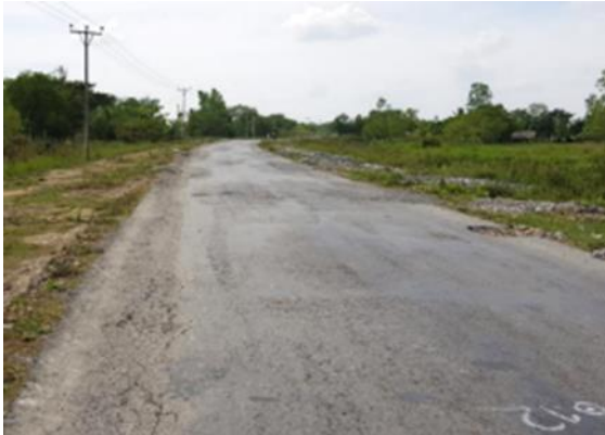
Figure 30: Site before trial
