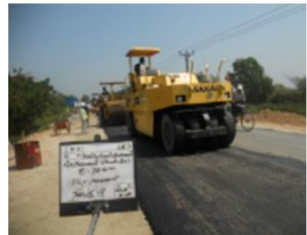
Figure 29: Secondary rolling
