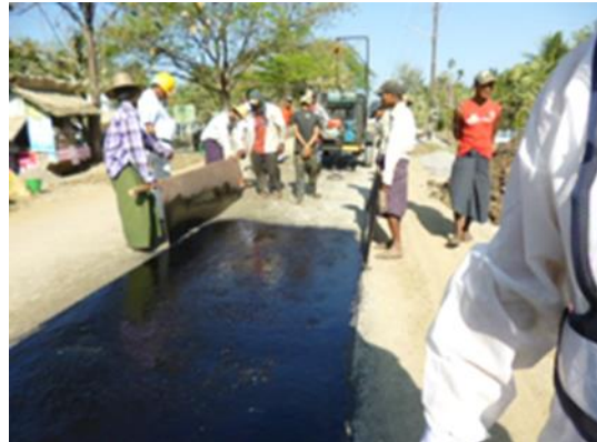
Figure 13: Laying bitumen
