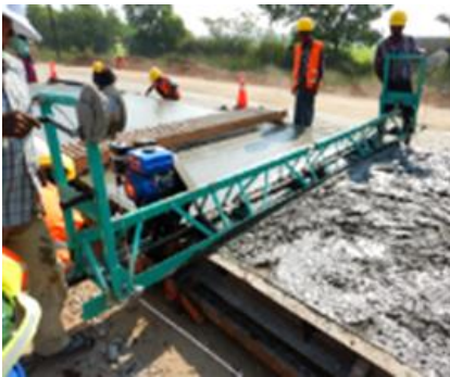
Figure 44: Manual finishing
