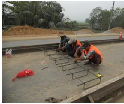
Figure 42: Installing the dowel bars
