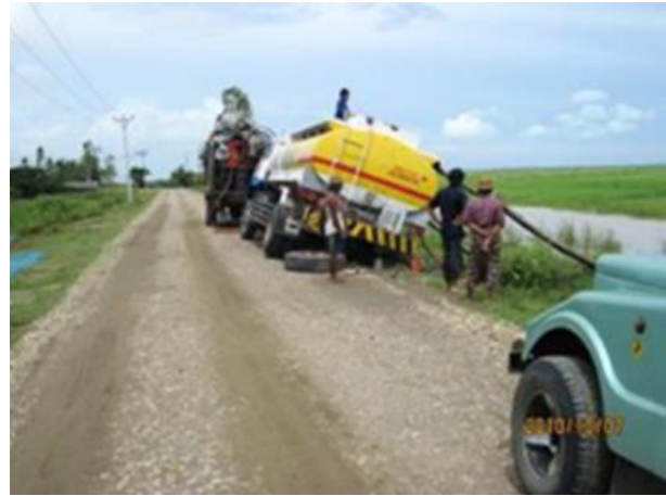
Figure 4: Damaged roads in rainy season (2010)
