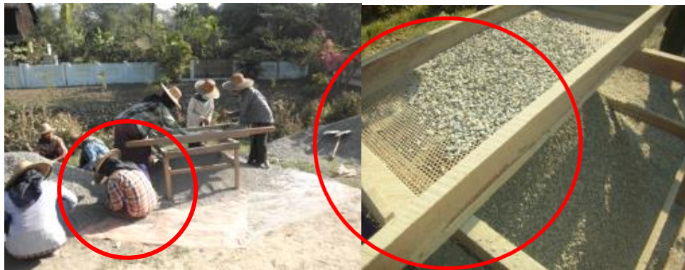
Figure 9: Preparation work (materials preparation)
