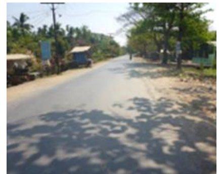
Figure 19: Pavement 4 years after construction (2018)
