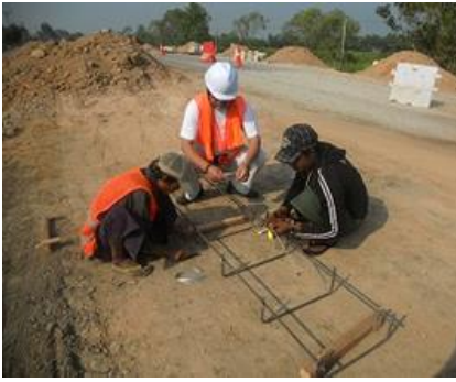
Figure 41: Assembling the dowel bars
