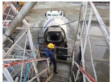
Figure 37: Adding water to the mix
