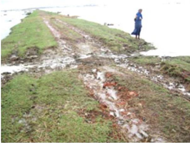
Figure 3: Normal condition of a rural road
