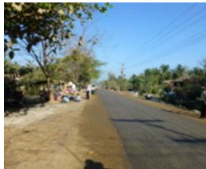
Figure 18: Pavement just after construction (2014)
