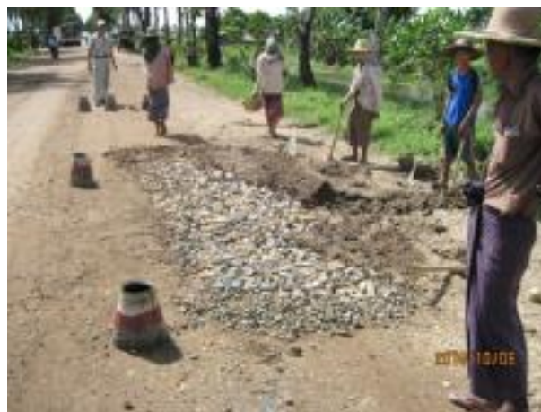
Figure 5: Damaged roadway after flooding
