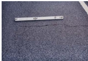
Transverse cracking
