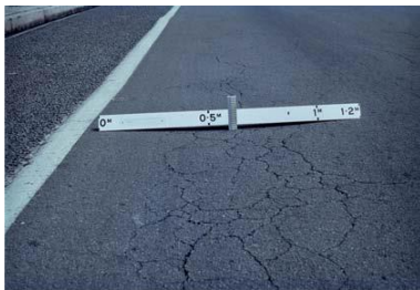
Crocodile cracking
