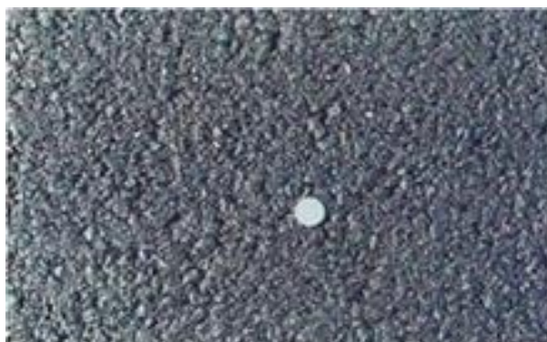
Figure 3-10: Gap-graded asphalt
