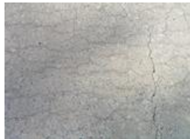
Alkali aggregate reaction
