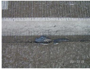
Joint spalling
