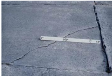
Fatigue cracking
