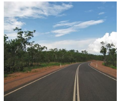
Sprayed/chip seal pavement – Australia
