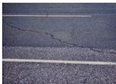
Diagonal cracking
