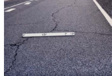
Block cracking
