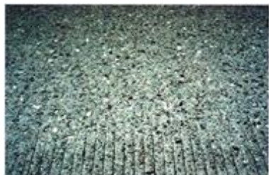
Abrasion or ravelling by studded tyre
