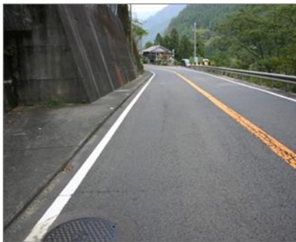
Asphalt pavement – Japan
