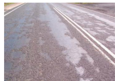
Stripping of sprayed seals
