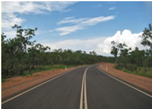
Figure 3-13: Typical sprayed/chip seal surfacing
