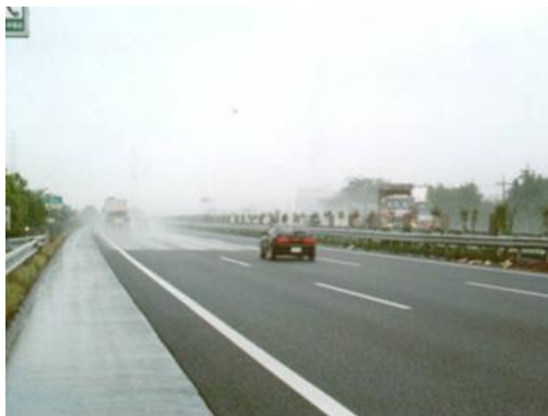
Figure 3-8: Porous asphalt
