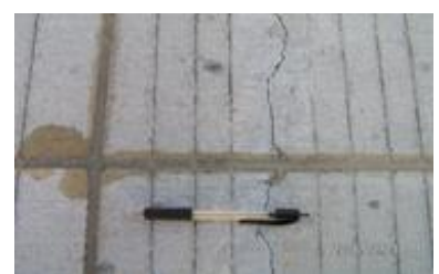
Transverse cracking
