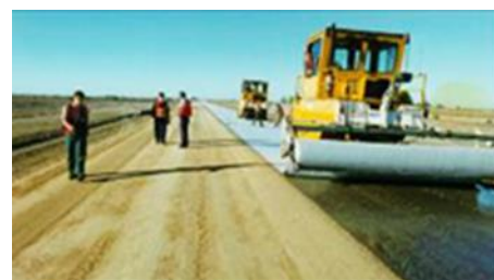
Figure 3-15: Geotextile reinforced seal pavement
