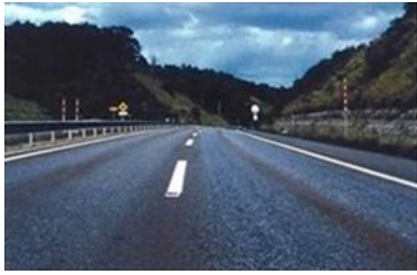
Abrasion or ravelling by studded tyre
