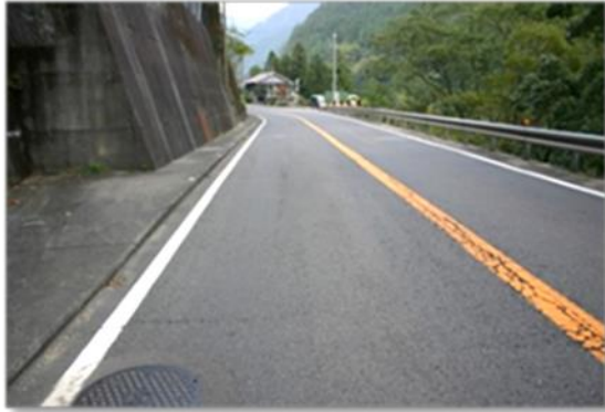
Figure 3-7: Dense-graded asphalt
