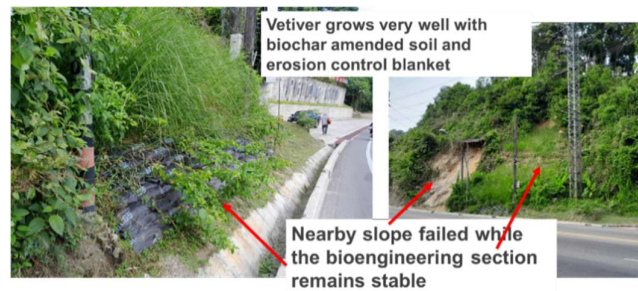
Figure 5: Bioengineered slope with vetiver and biochar in Phuket province
