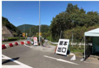
Operation of the gate at Sakamoto PA (outbound)
