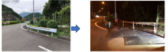
Before and after installation of the gate at Sakamoto PA (outbound)
